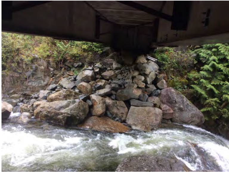
Left Bank Abutment when facing downstream
