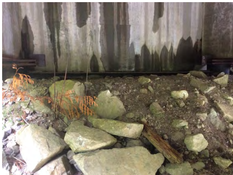
Right Bank Abutment when facing downstream
