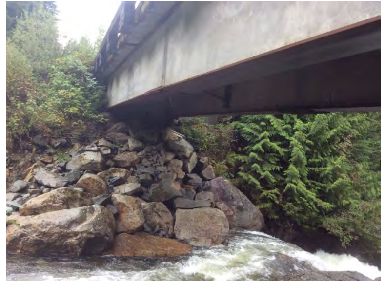
Left Bank Abutment when facing downstream
