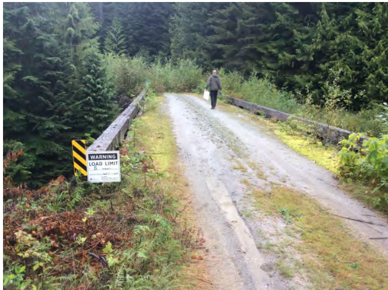
Load Rating Sign
